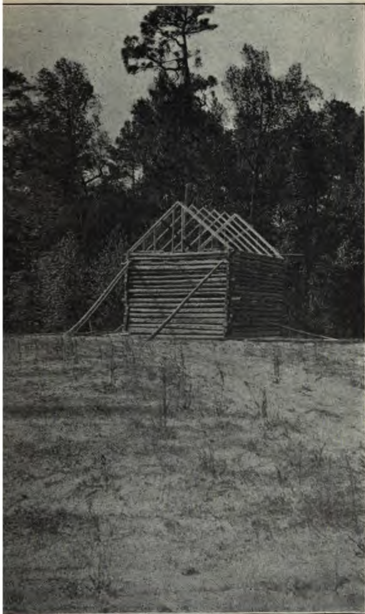
LOG BARN FOR FLEE CURING, IN PROCESS OF CONSTRUCTION.
