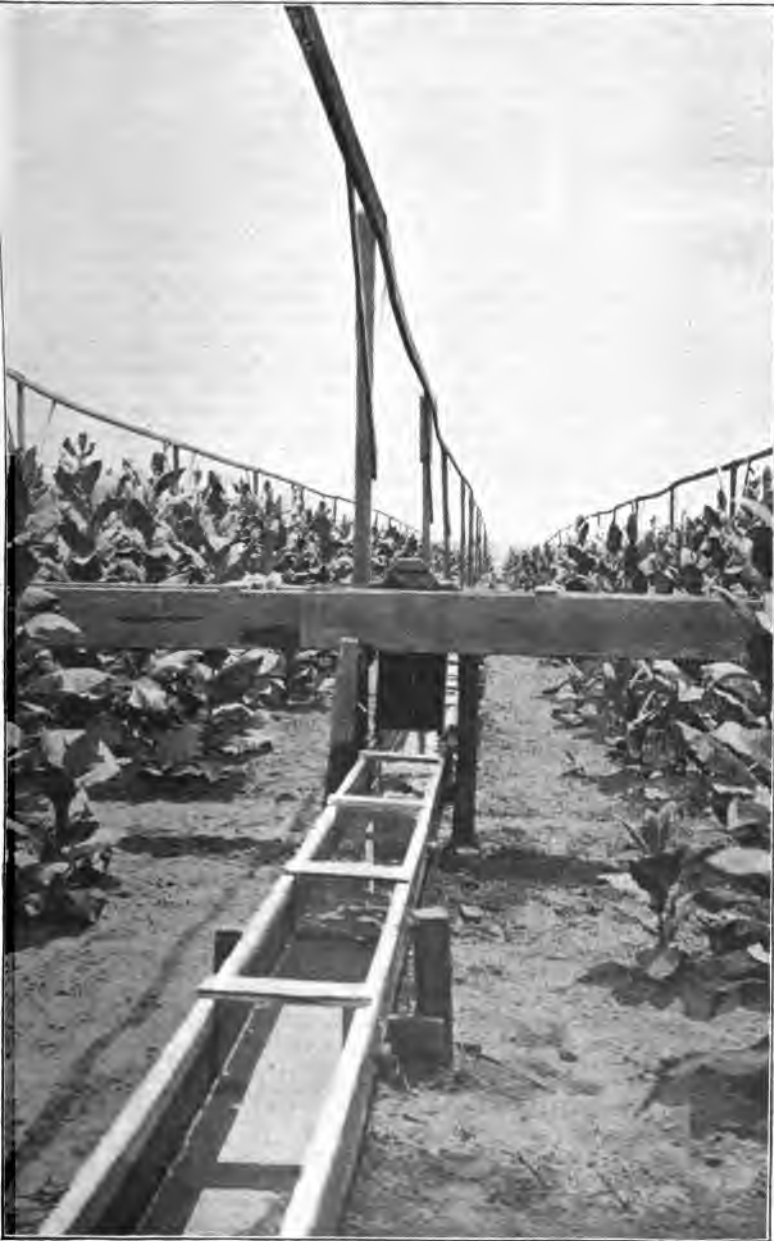
SHADED SUMATRA TOBACCO, SHOWING SYSTEM OF FLUME IRRIGATION. K2
